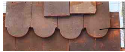
Proposed sample board of tile hanging and roof tiles at plot rear of 6 Somerset Way
